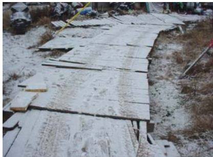
"New" Boardwalks made from discarded wood
