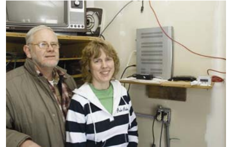
Gavin & Judi Thompson of Dillingham stands next to a radio unit
